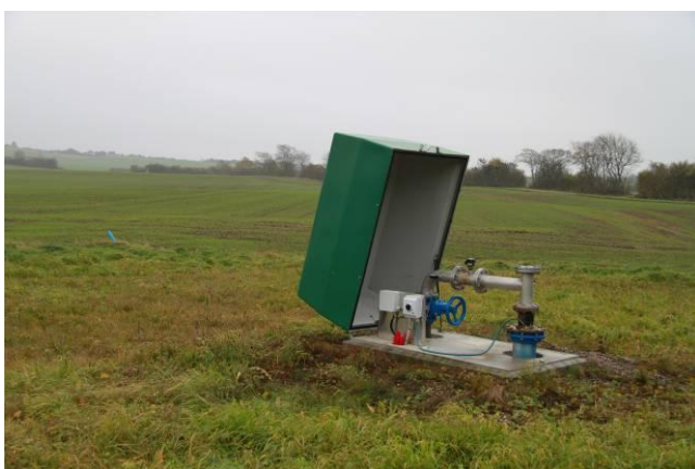
Figur 5 Mjang Dam boring 170.315
