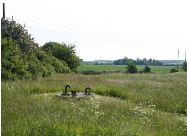
Figur 4 Mjang Dam boring 170.320
