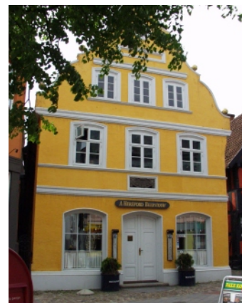
Flot istandsat facade.
