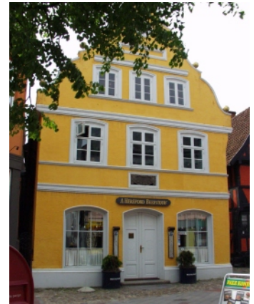
Flot istandsat facade.
